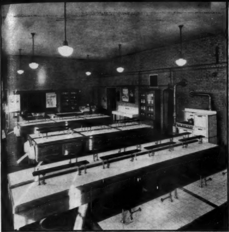
BEFORE Langley High School's domestic science classes were held here—clean and neat, yes, but entirely lacking in the concept of modern home life in relation to arrangement and use of time-saving domestic equipment and today's electrical way of living.
